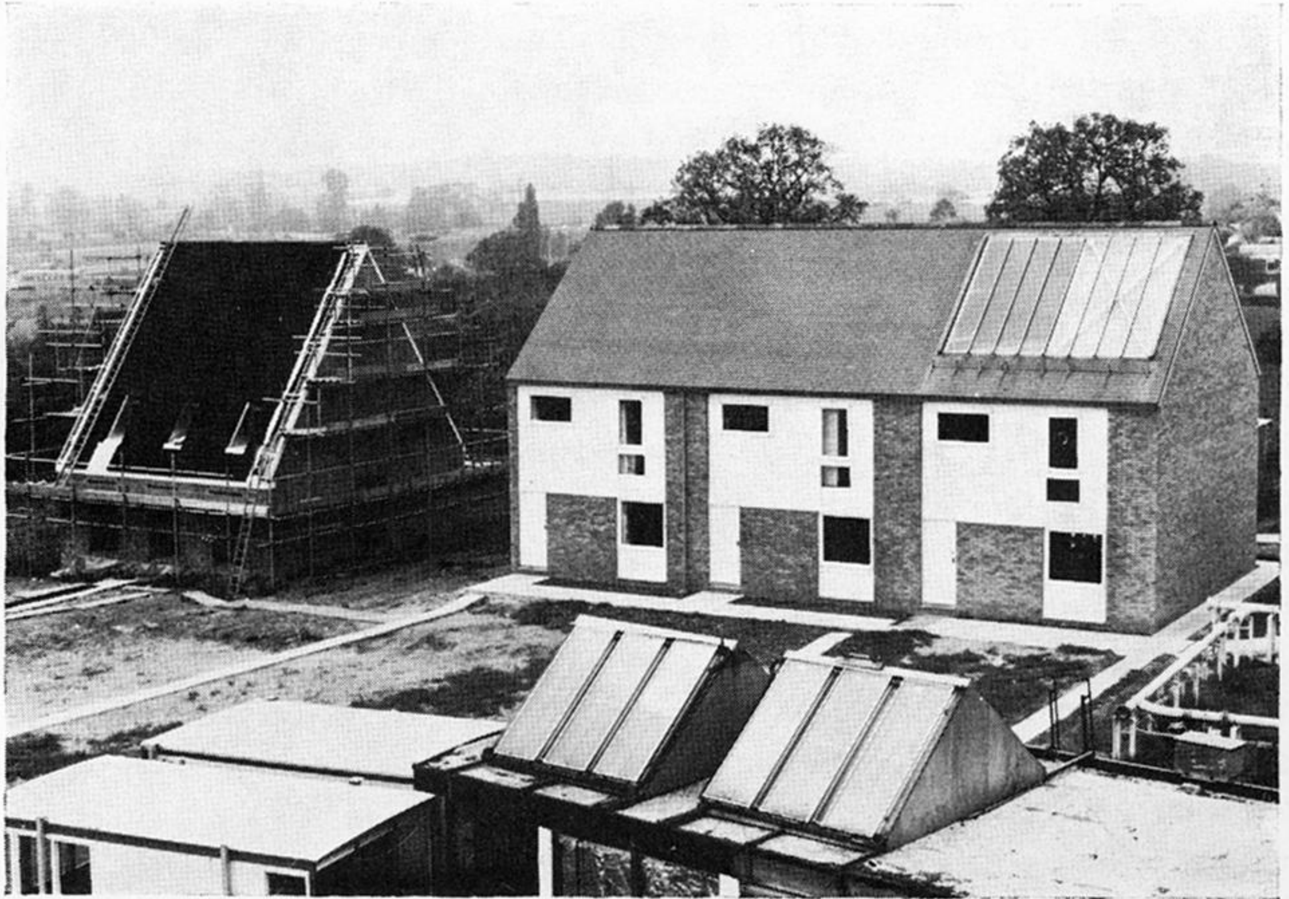
FIGURE 5. Four experimental low energy house laboratories at the Building Research Establishment.
